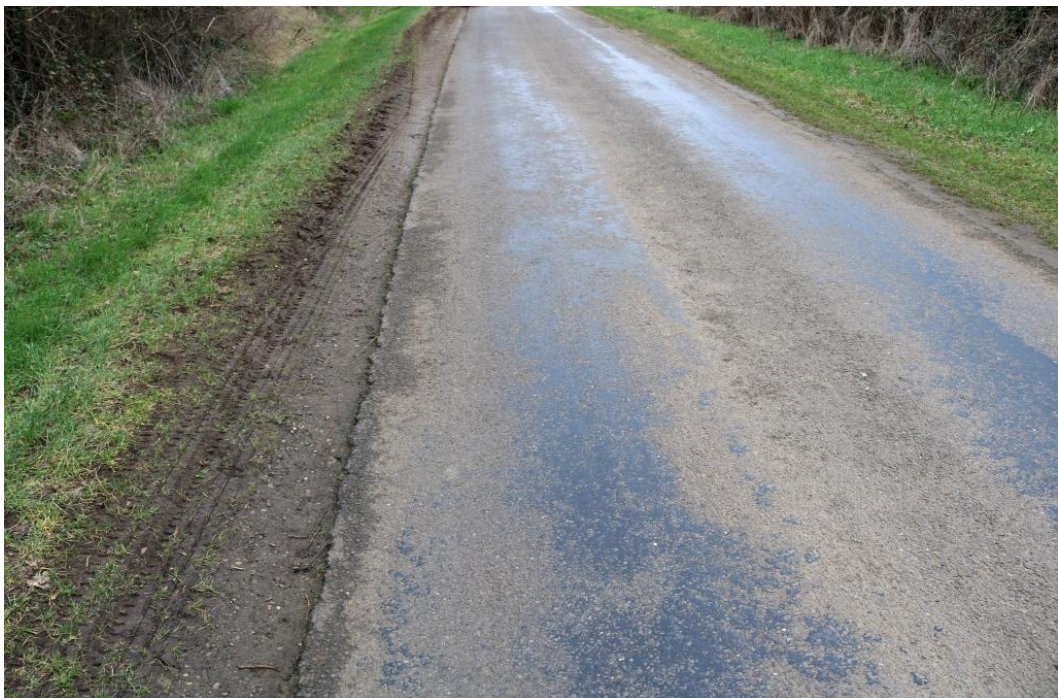
Damage to verges along Uffington Lane
